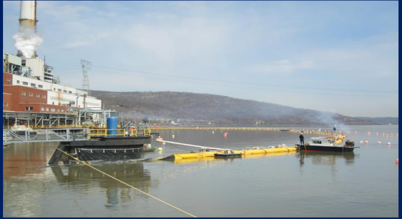
Figure 3. Installation of the Lovett BSFB MLES
