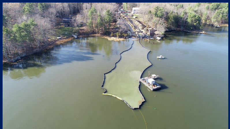
Figure 5. Drone footage of barrier during hand jetting operations
