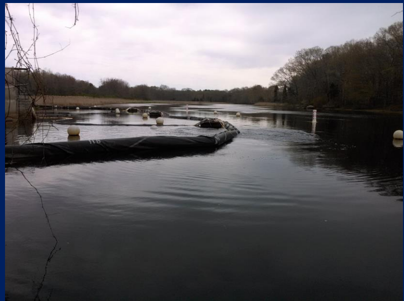
Figure 4. Side view of barrier system in Taunton River
