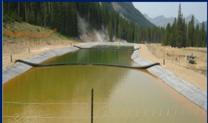
Figure 2. Aerial view of deployed barrier system
