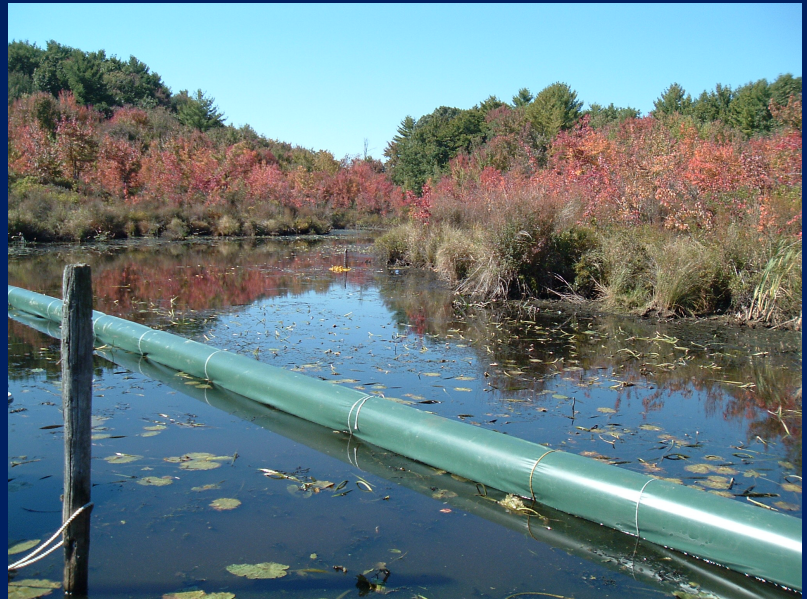
Figure 3. Boom installed across the Back River
