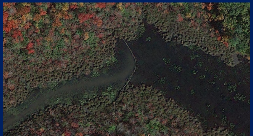
Figure 2. Aerial view of upstream barrier vs downstream barrier
